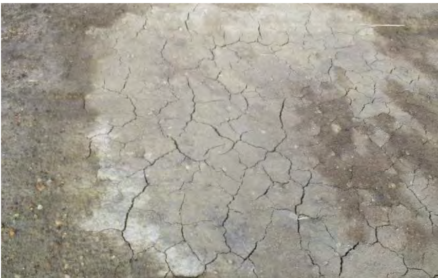
Photograph showing a closer view of soil cracks with slight salt crusts on site.
