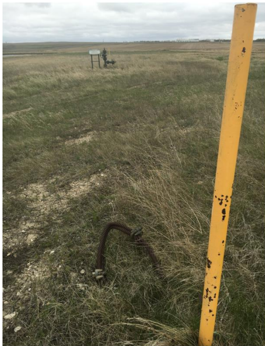
Figure 8: Wellhead and above grade infrastructure, including the cable, rig anchors, and postings.
