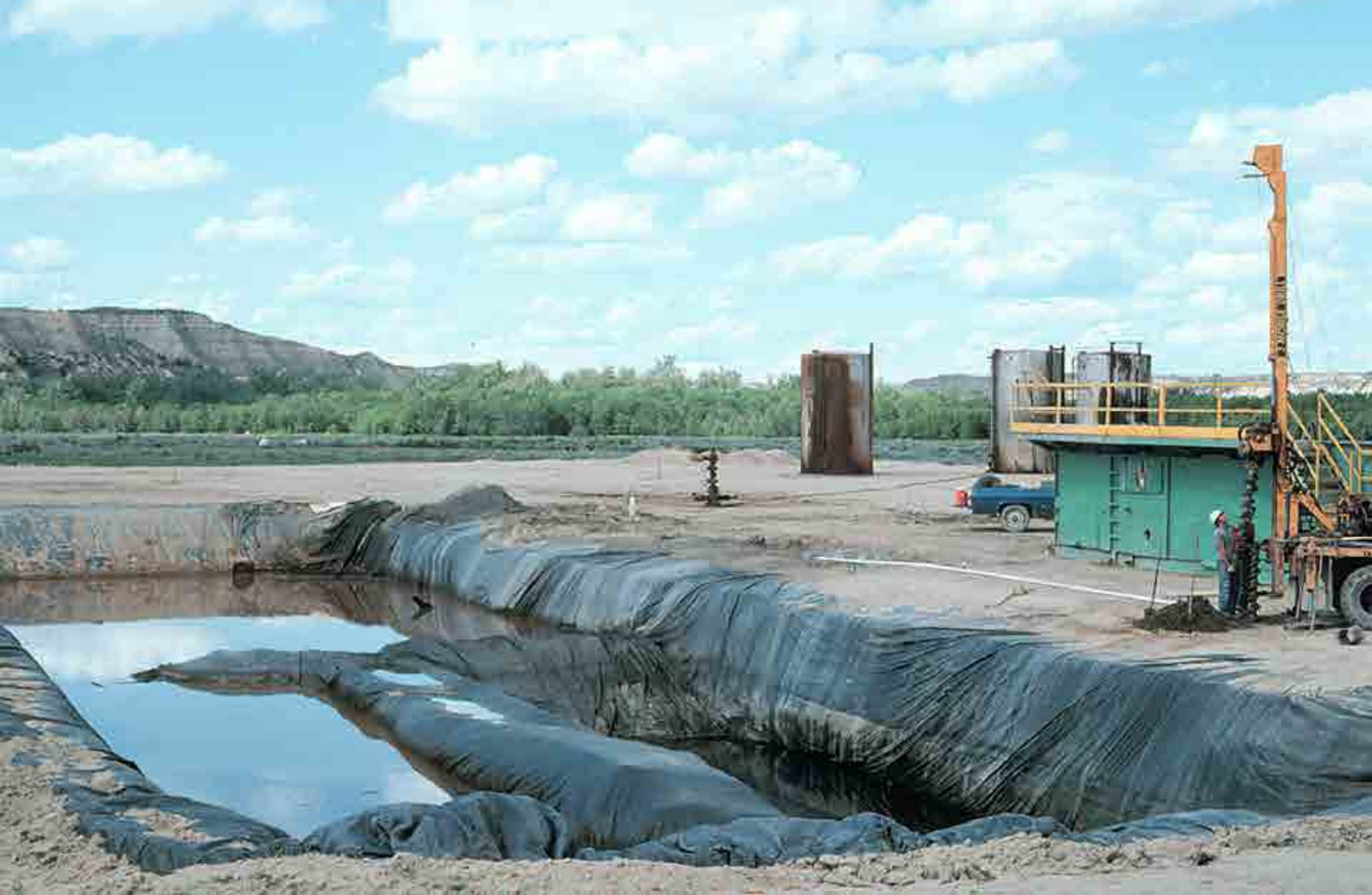
APACHE FEDERAL 1-5 Installing monitoring wells in 1981.
