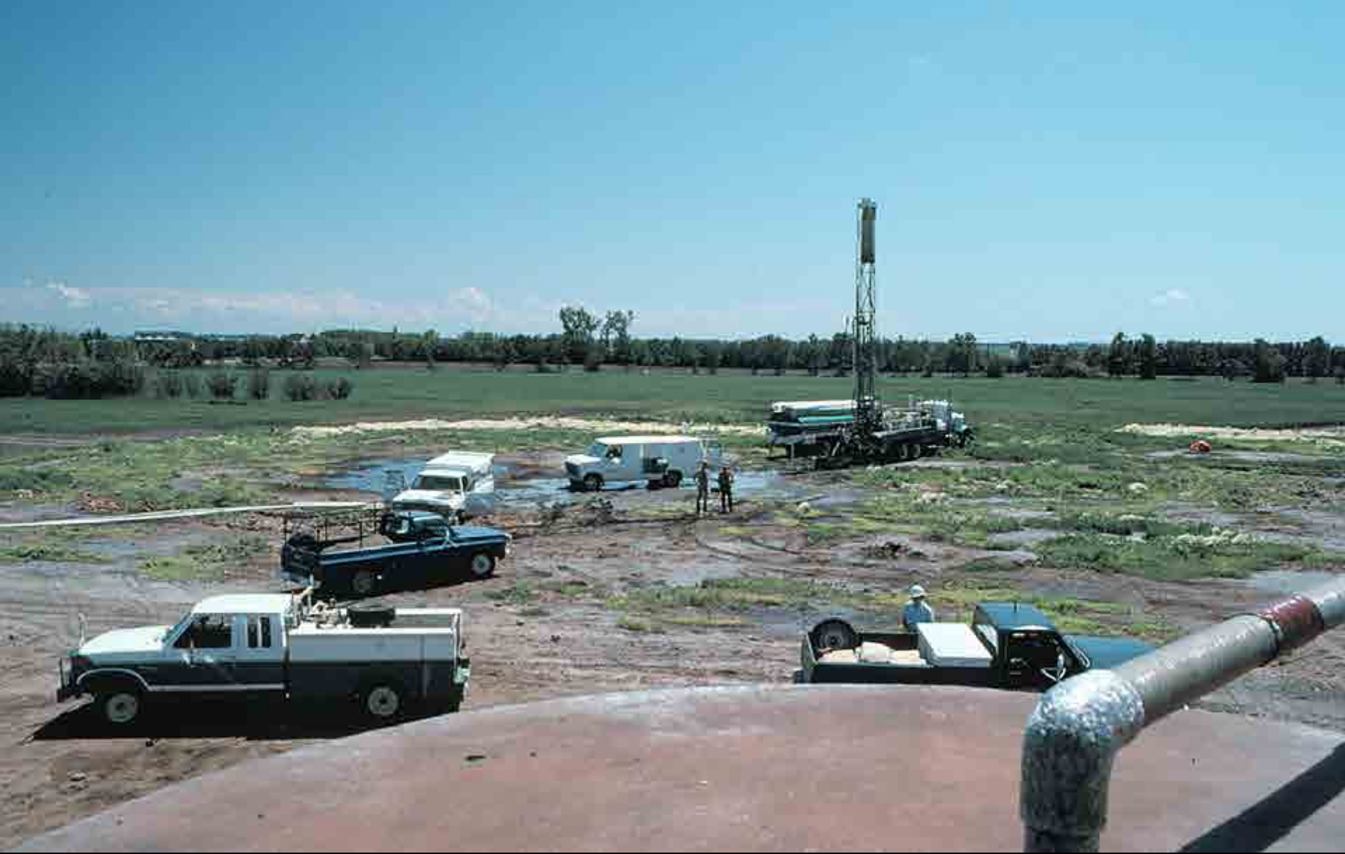
Installing monitoring wells at the Stratton SWD #1 in 1984.
