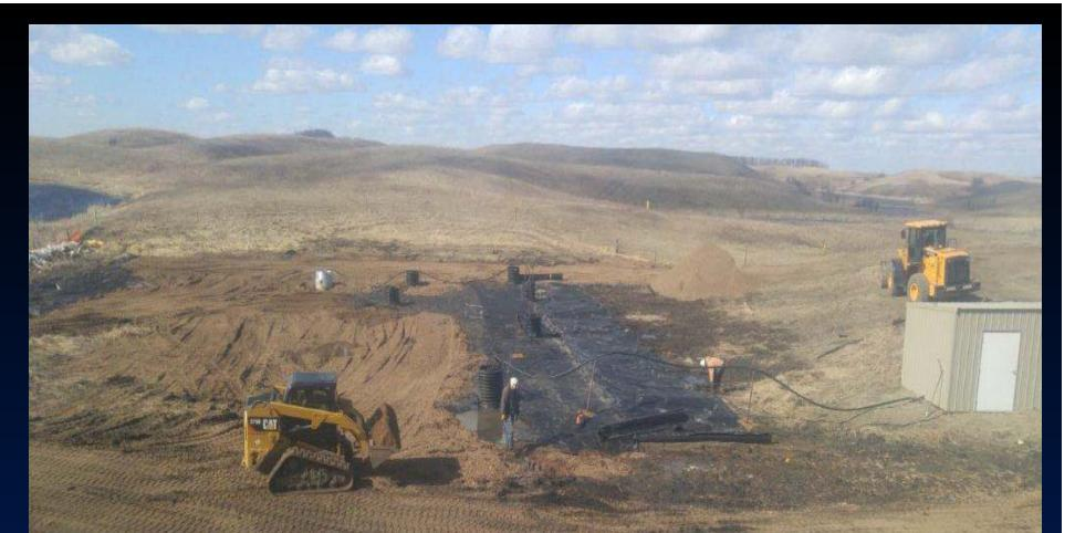
Area was covered with geofabric, geogrid, and cover rock to confine the contaminated soil and create a firm working surface. Surface materials were removed at completion.
