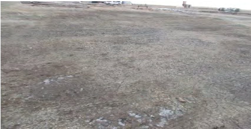
Photograph facing west showing a closer view of the cracking soils at the visually impacted area located within the laydown yard of the oil & gas facility.
